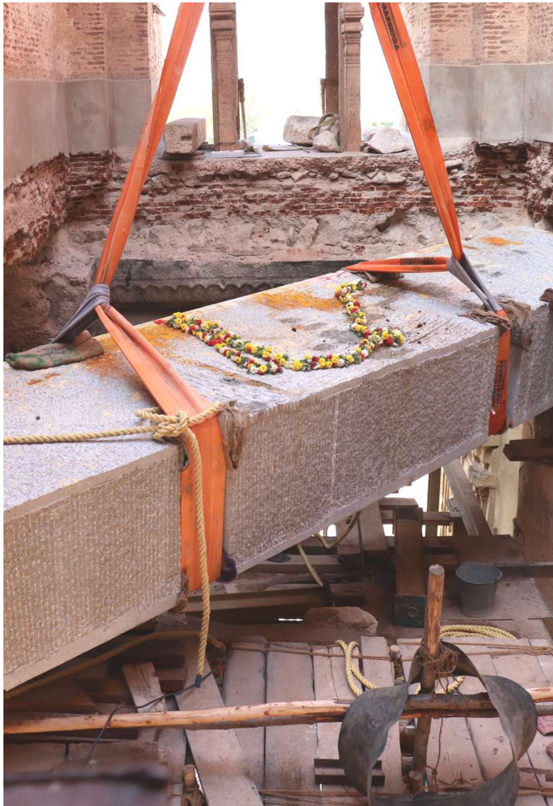
Shree Pundarikatcha Perumal Temple - Thiruvellarai Renovation work - Jan 2020
