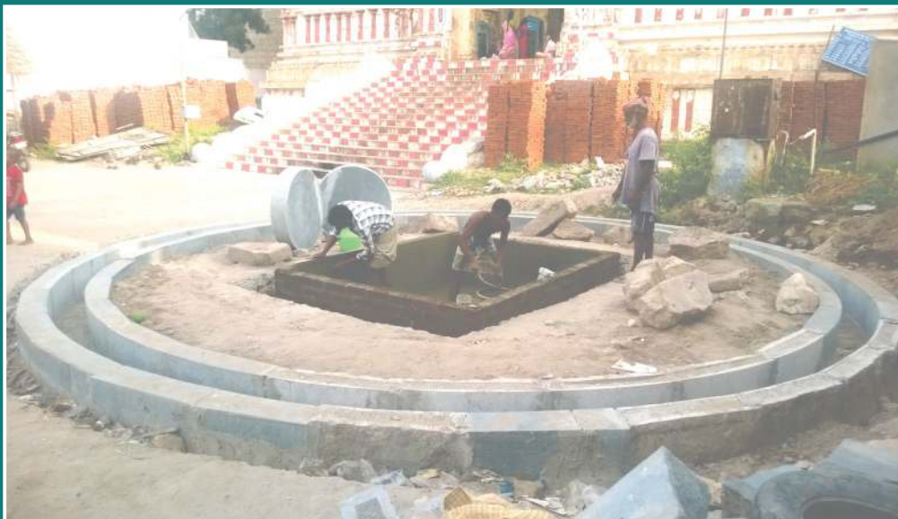
Traditional Lime-Mortar preparing arrangement in construction phase
