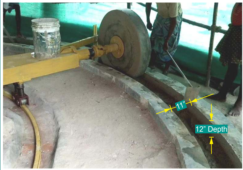
Another view of the Lime-Mortar mixer
