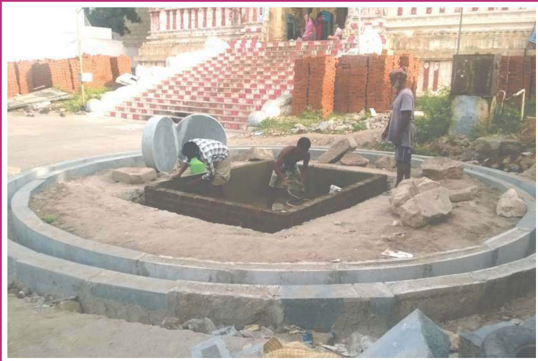
Traditional Lime-Mortar preparing arrangement in construction phase
