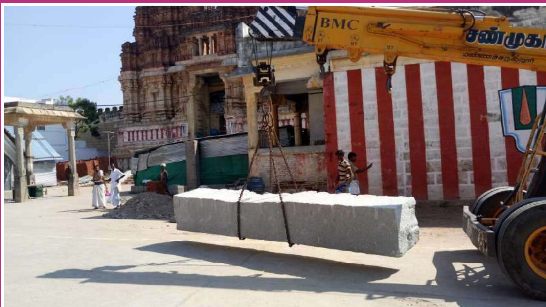
The first set of beams arrived at the temple on 9 Feb 2017
