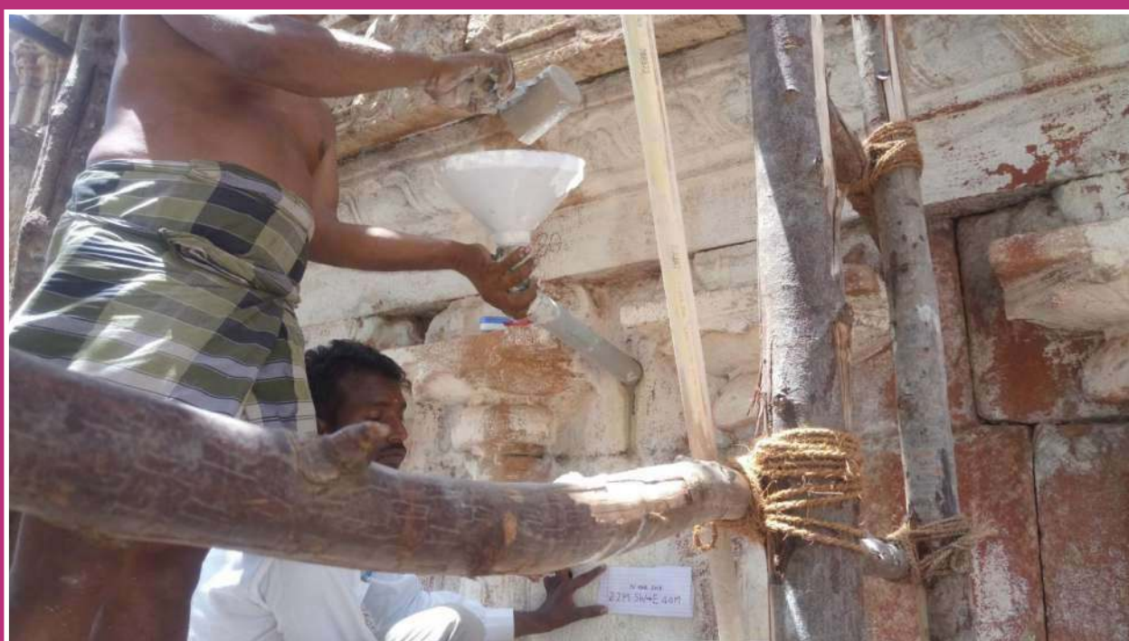
Injecting the Lime-Mortar Slurry
