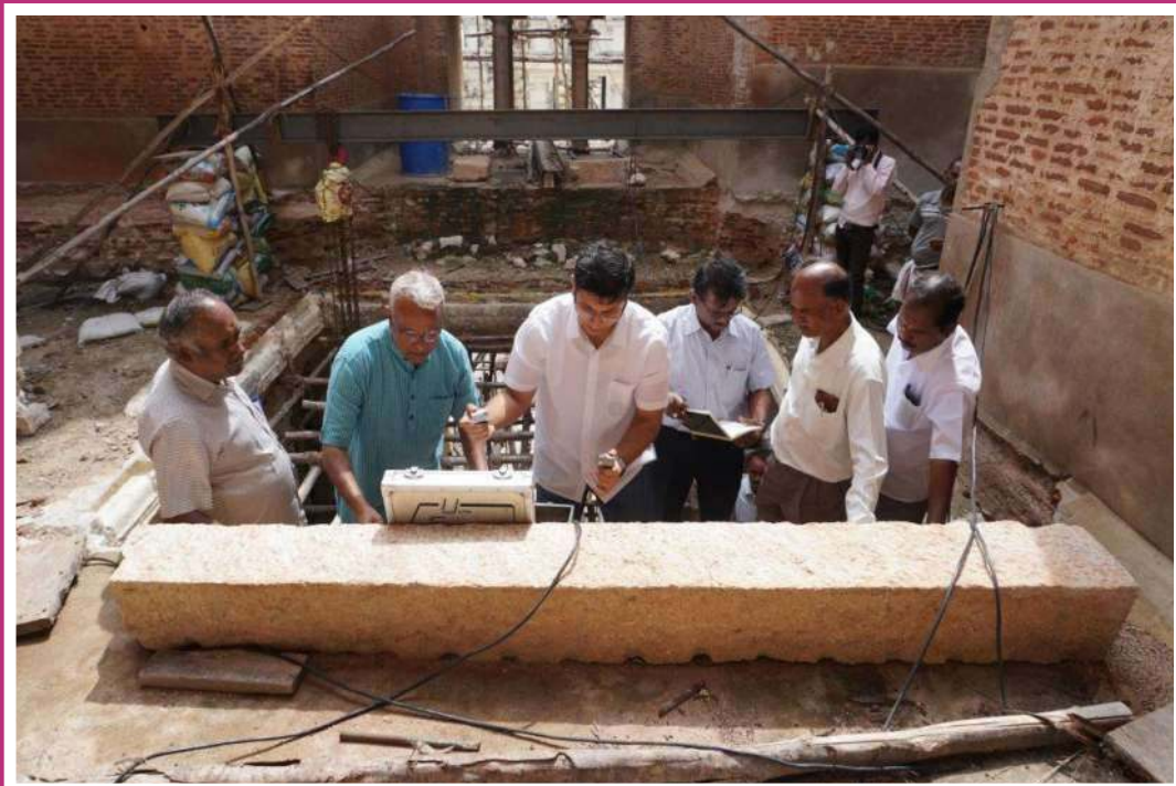
The team testing the granite beams (kathavadi) for cracks
