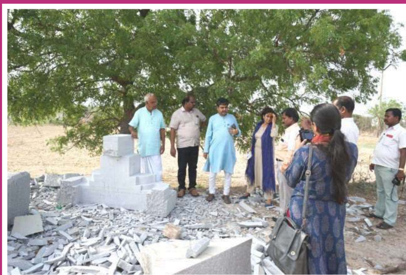
UNESCO & ASI team along with Joint Commissioner inspecting the work in progress
