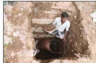
Figure 5: Trial pit at location 2 in progress
