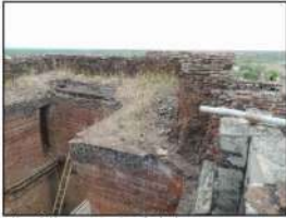
Figure 2: Masonry section above first level
