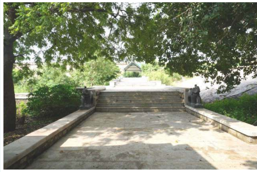
South prakaram - Western side Jul 2016
