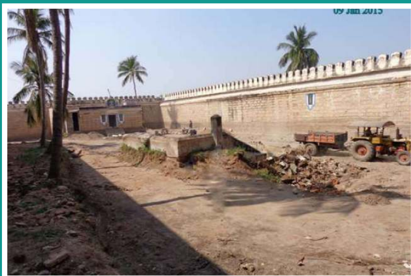
North prakaram - During renovation Jan 2015
