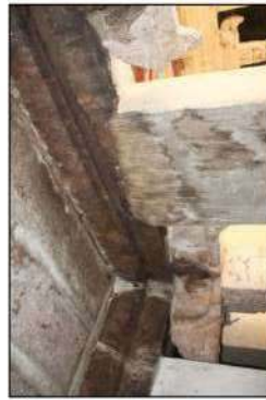
Figure 8: Masonry section inferred with bars
