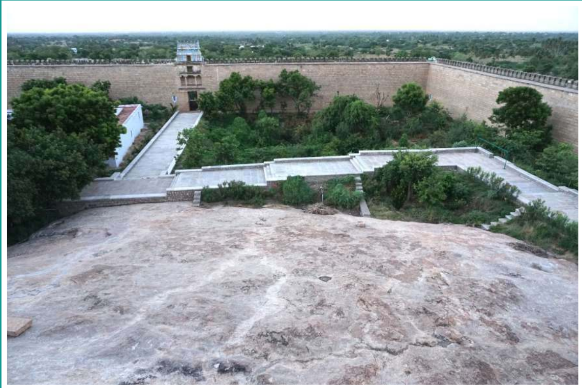
South west prakaram - After renovation Mar 2016
