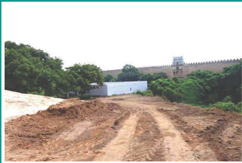
South west prakaram - During renovation Nov 2014
