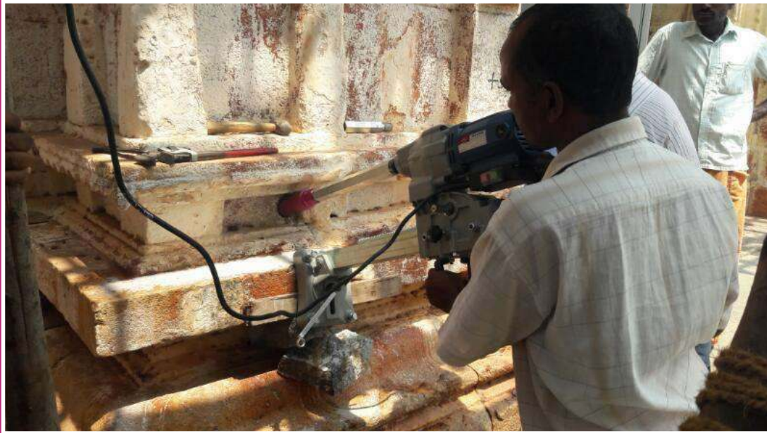
Core drilling in progress
