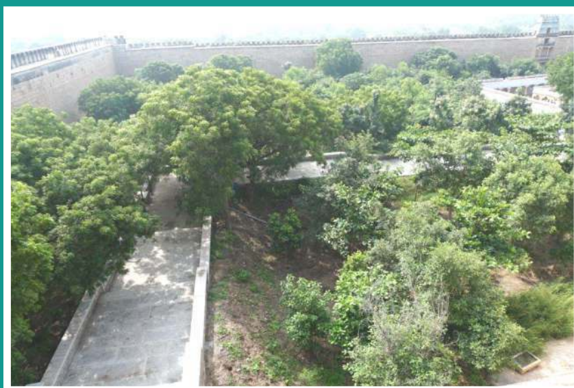
South east prakaram - After renovation Nov 2016
