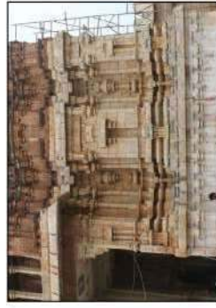
Figure 10: Cracks on granite beam and temporary support system
