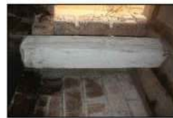
Figure 12: Masonry pier as temporary support
