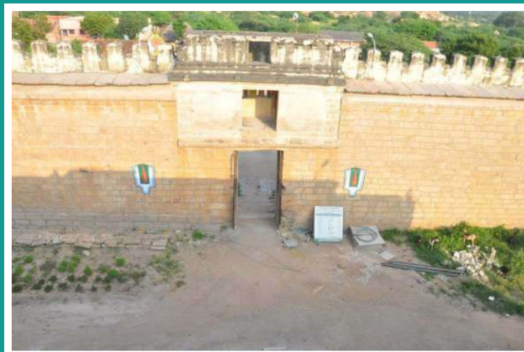
Eastern entrance - During renovation Jan 2015
