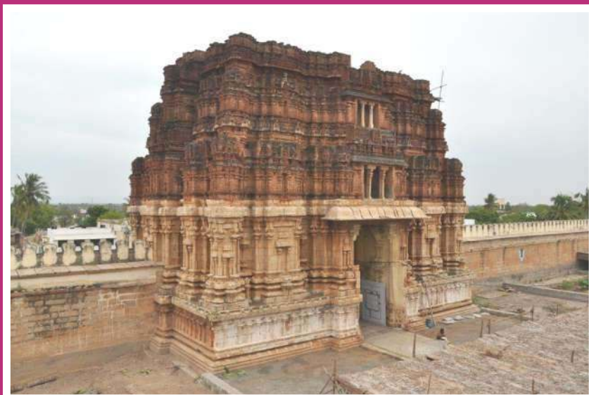
View of the Raja Gopuram from Northwest part of 4th prakaram
