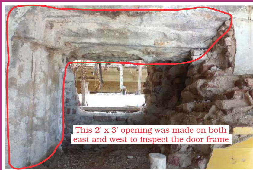
Damaged door frame
