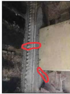
Figure 4: Deteriorated timber members
