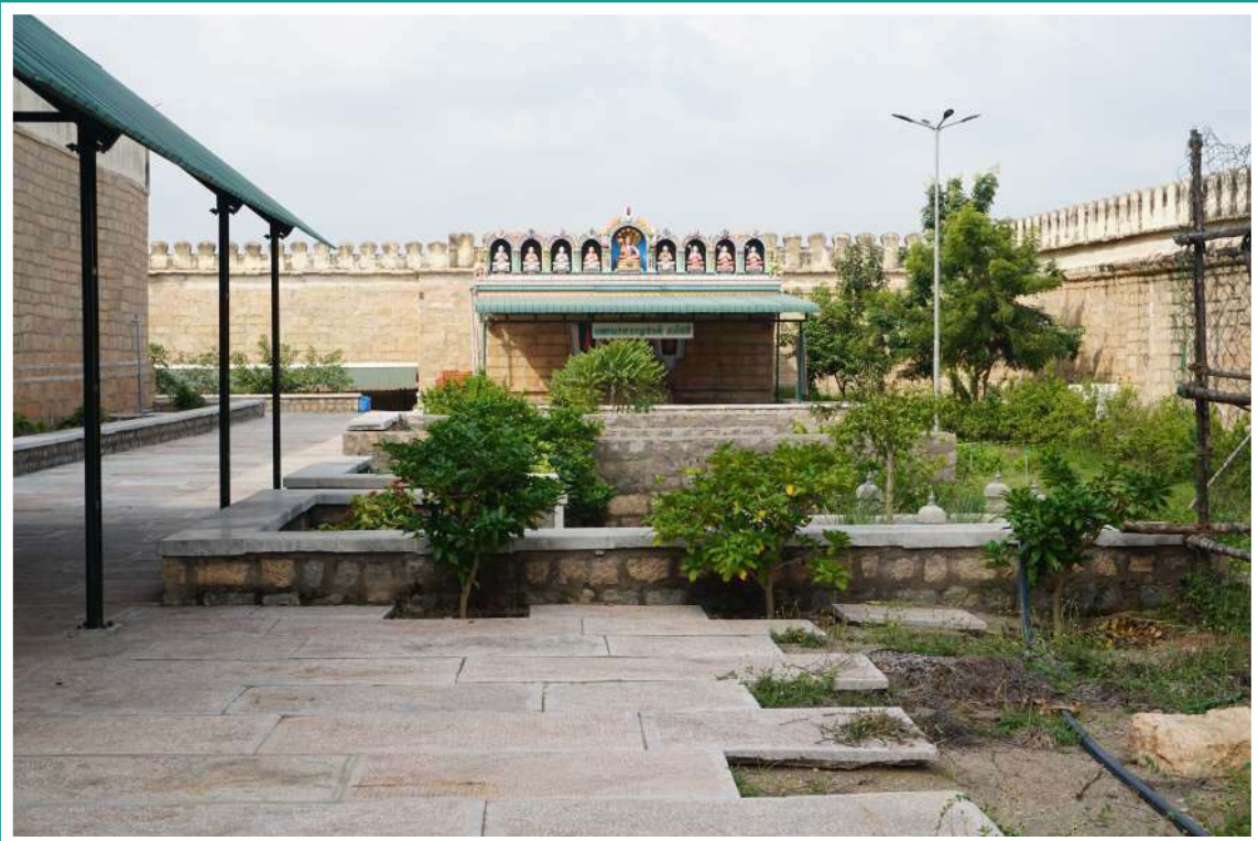
Manavala Mamunigal Sannidhi After renovation Dec 2016
