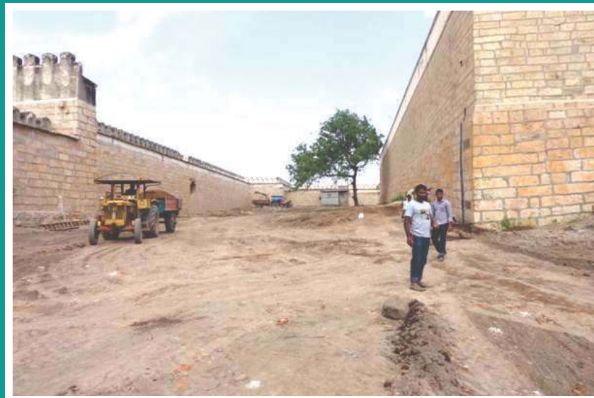
Southwest prakaram - During renovation Oct 2014
