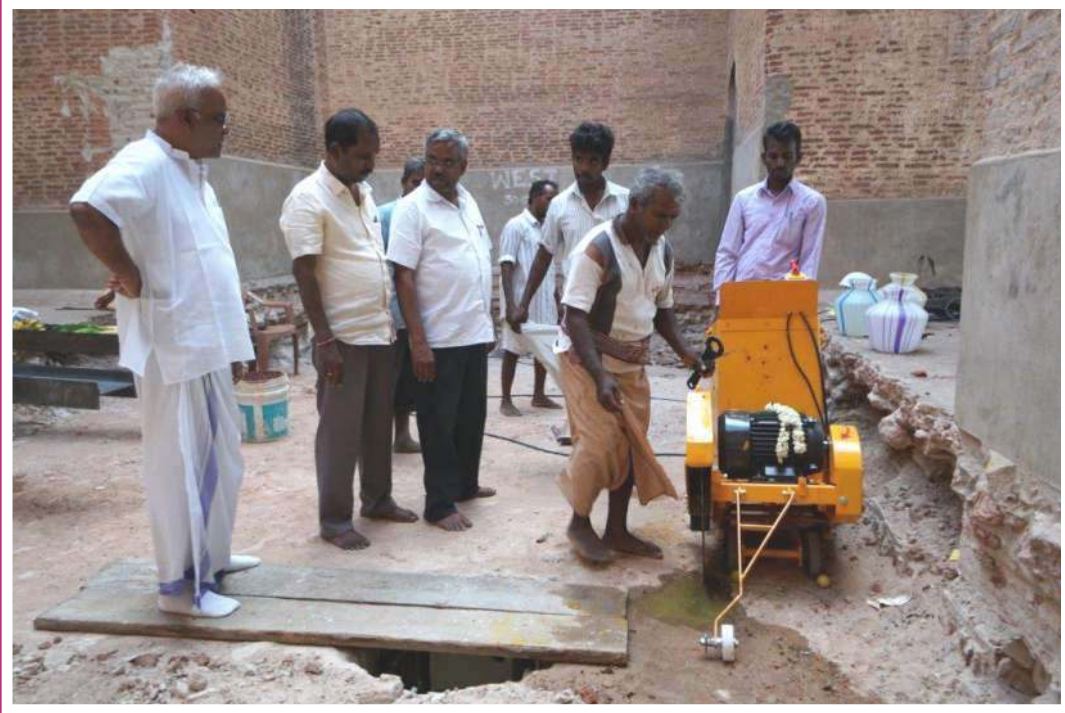
Core cutting process in action
