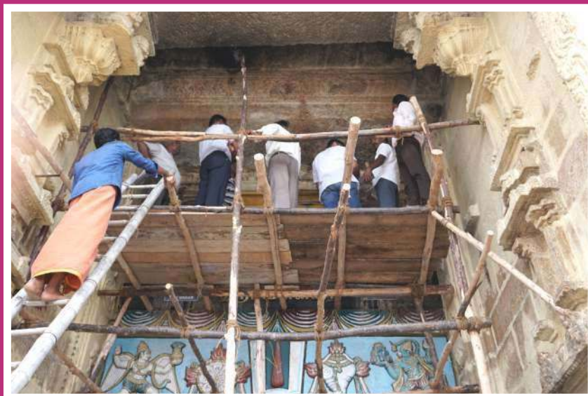
Inspecting the door frame at the entrance
