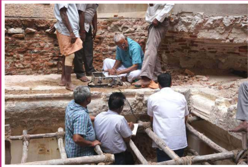
Kathavadi granite beam
